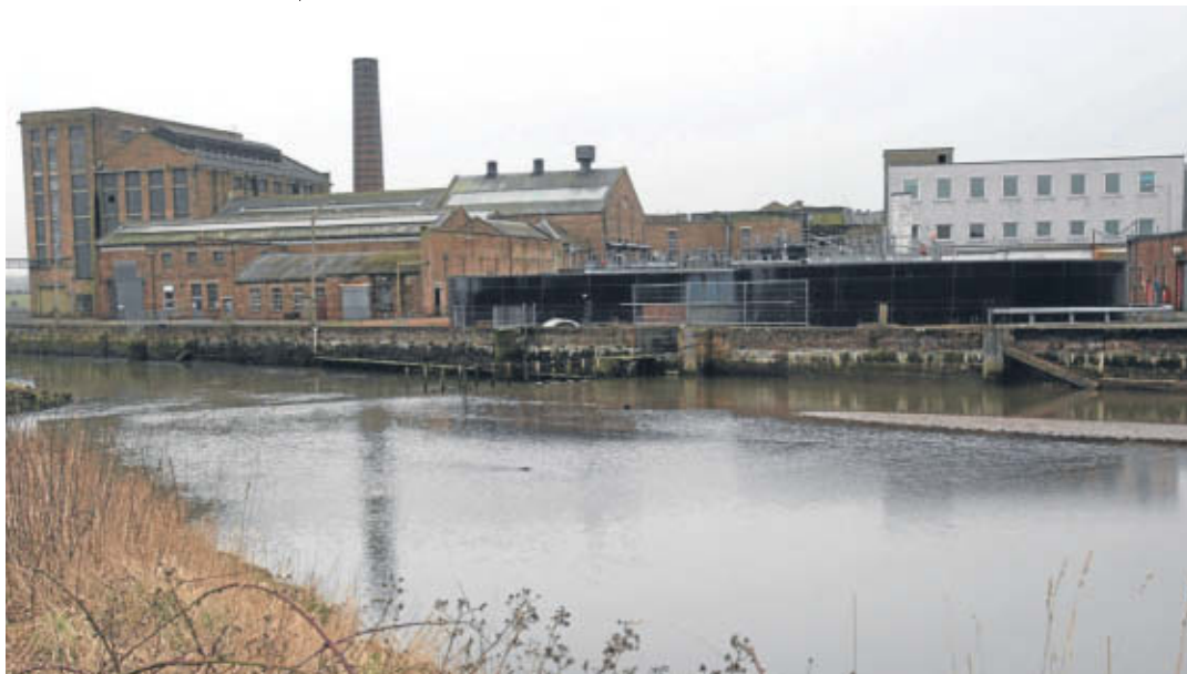
The former paper mill at Guardbridge which now houses St Andrews University's energy centre.
